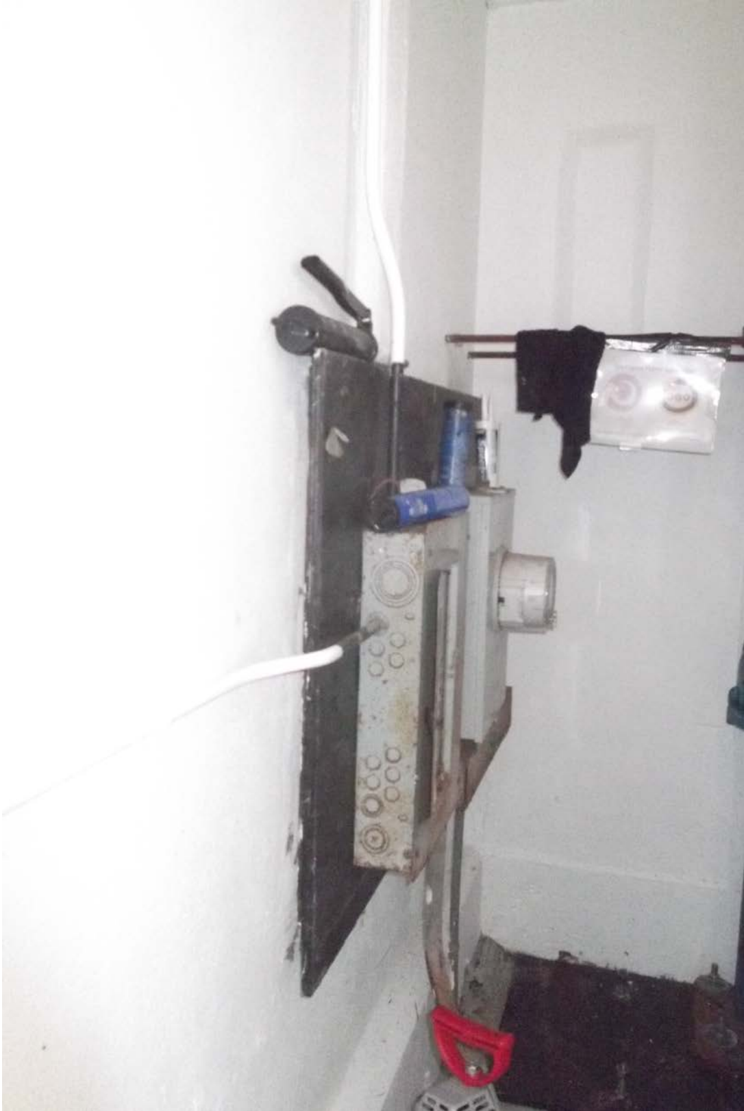
Existing Electrical Service to be Removed & Raised
